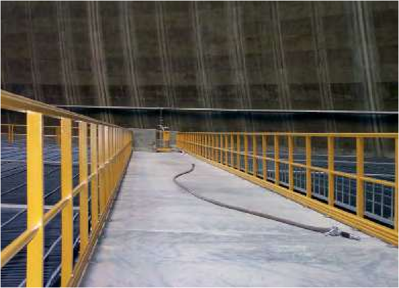
Top: GRP handrails on a cooling tower
