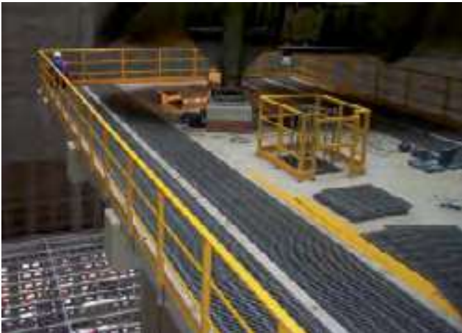
Top: GRP handrails on a cooling tower
